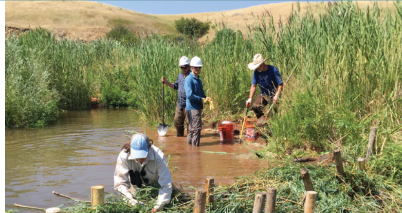
Building beaver dam analogs helps restore wet meadows on western rangelands. Photo: Mandi Hirsch.
